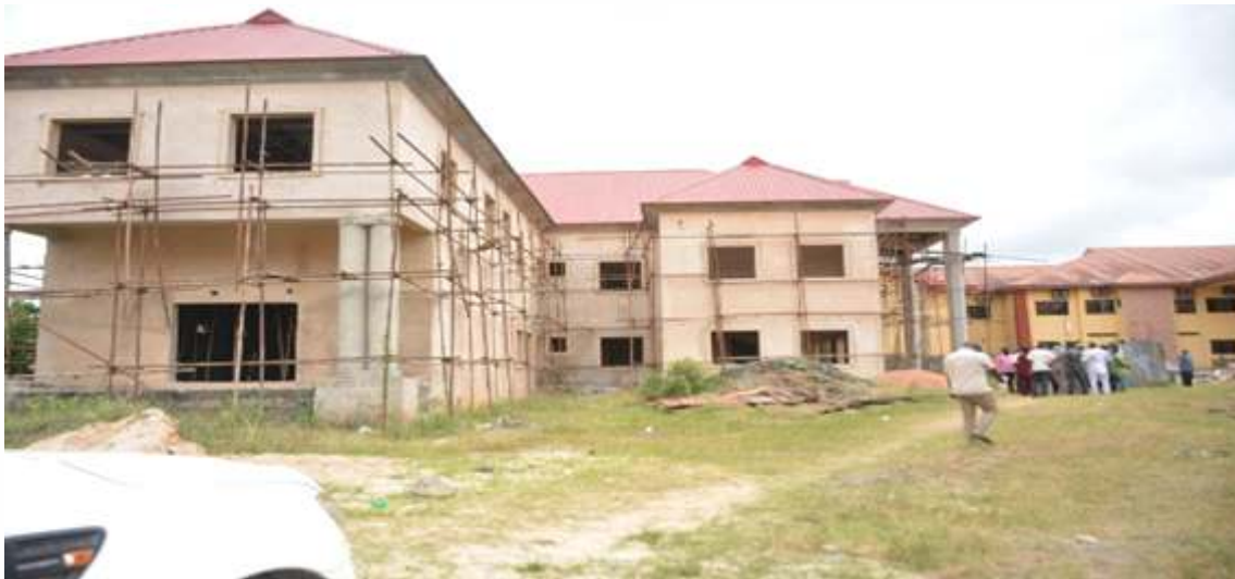
On-going Magnetic Resonance Imaging (MRI) Building at FMC Owerri, Imo State
