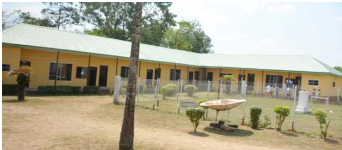
Complete Rehabilitation of Classrooms at Federal School of Forestry, Ibadan
