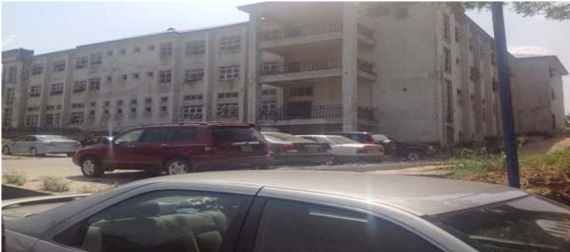
The two-storey Renal Dialysis, ICU Building at FMC, Asaba
