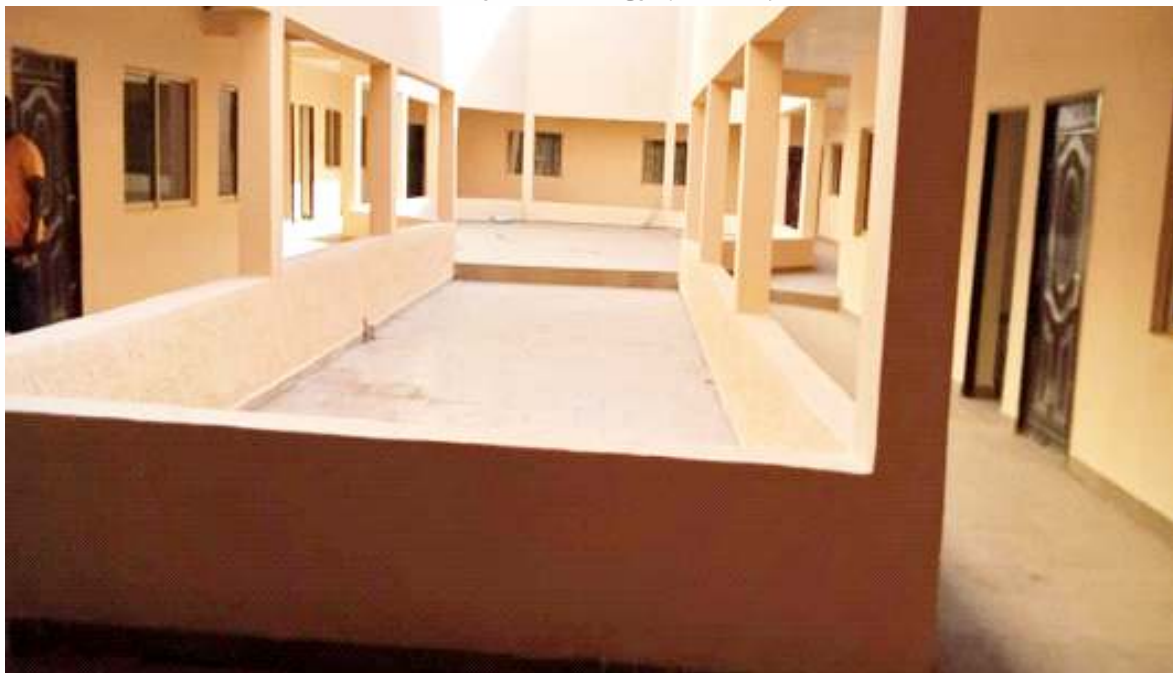
Courtyard of classroom block at Police intelligence School Share, Kwara state.
