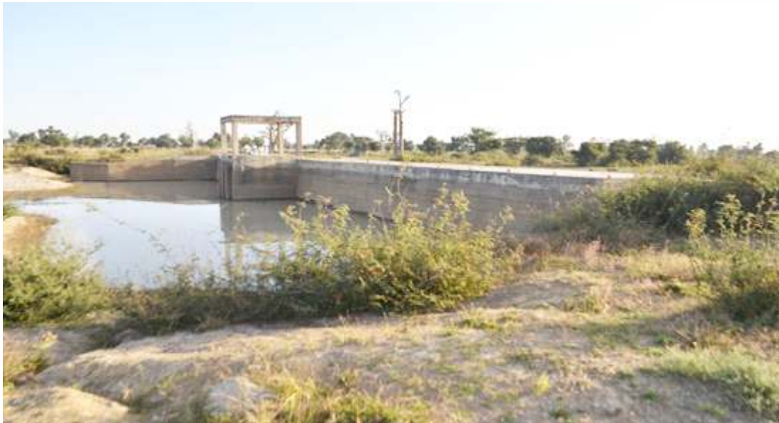
Construction of Gadau-Lafia/Zigau Earth Dam, Bauchi
